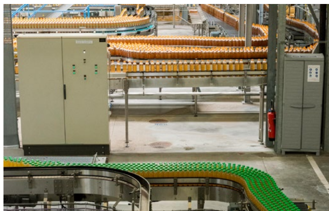
Plant bottling lines
